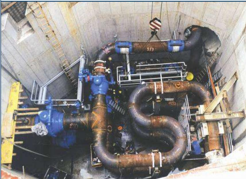
Ball valve model KHSVi & KHSVI fully welded
